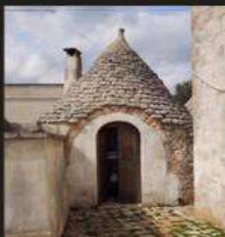
The trullo roof to be restored. The original stone shingles called chianche will be removed and replaced.
