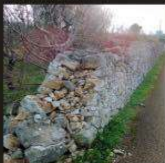
A typical dry-stone wall constructed of wild field stones in the Valle d'Itria area.
