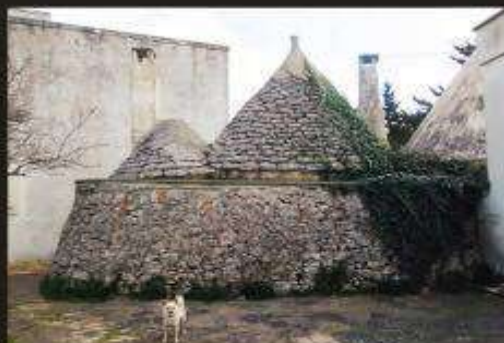
In addition to the roof restoration, there will be a stone stair constructed on the back side of the trullo to access the roof.
