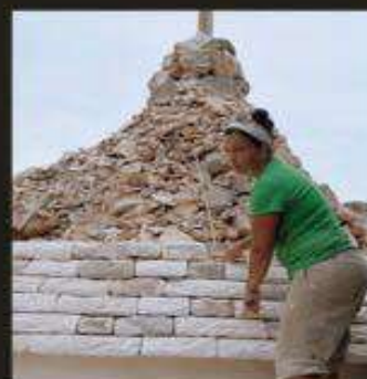
Thea Alvin instructing students on new and restored chianche placement on the 2014 workshop project.
